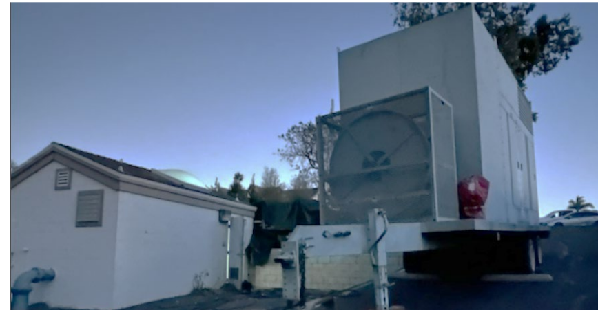
Second emergency generator being installed at Crestview office booster station
